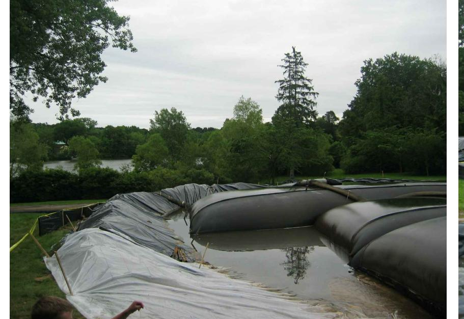
EXAMPLE GEOTUBE® CONTAINMENT AREA (HYDRAULIC DREDGING ONLY)
